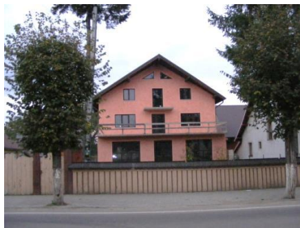
Fig.3: House of young couple that decided to build it on the plot of the wife's parents (author photo Marginea, 2010)
